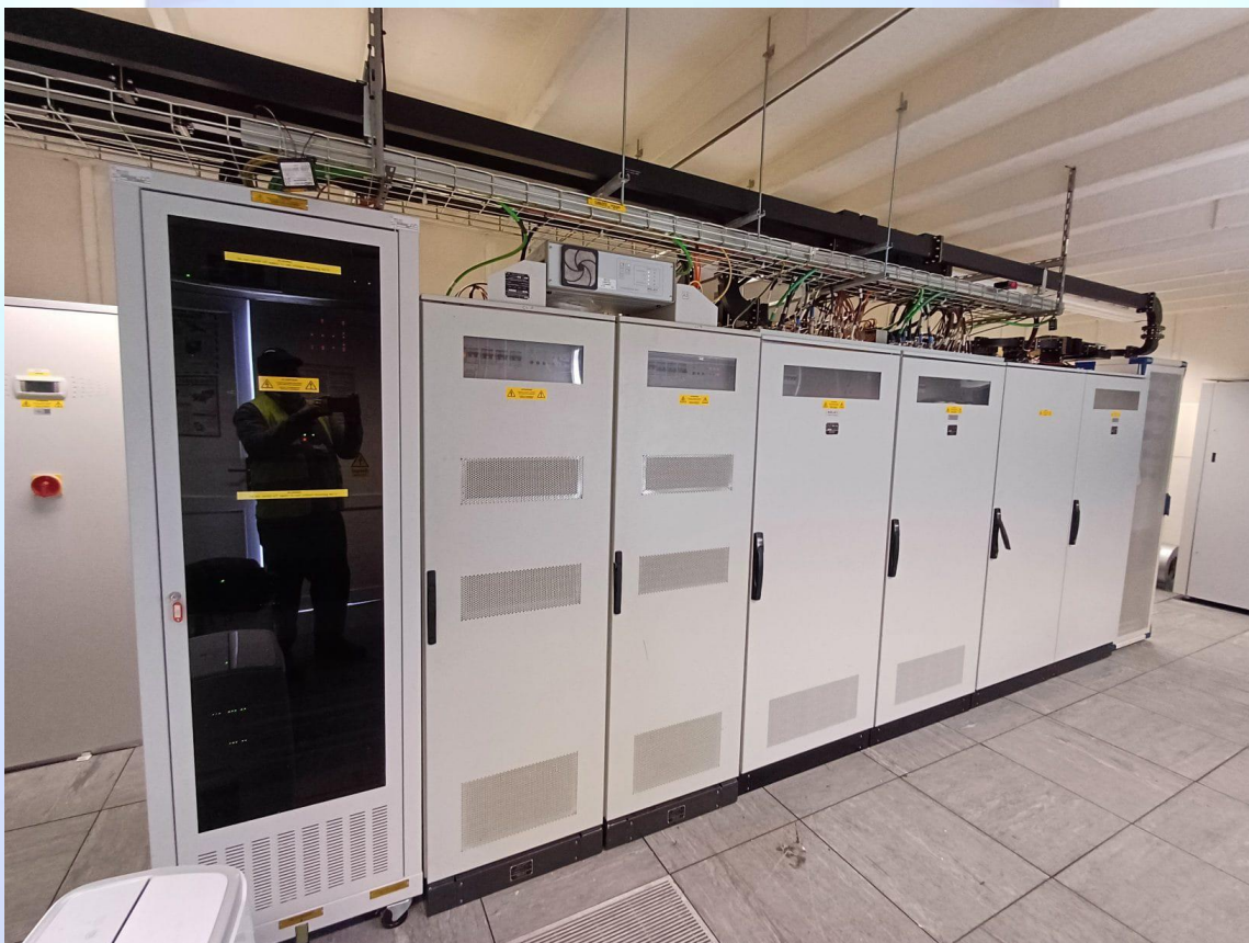
Radar system equipment racks illustrating core processing and signal handling infrastructure supporting operational performance and maintenance verification.
